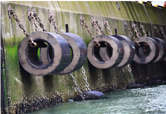
Figure 26: Fender configuration
