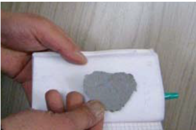
^ Loose rust scale will result in the hold failing the cleanliness survey
