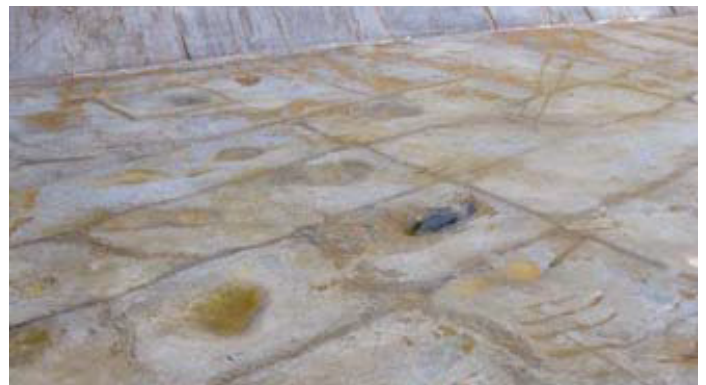
^ Check the tank top indents after discharge and after cleaning
