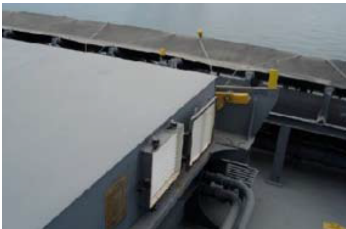
^ Maintenance of hatch cover vents is essential
