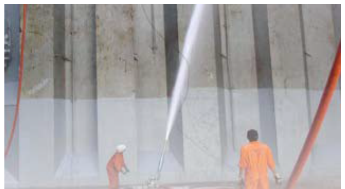
^ Hold cleaning using a maxi-jet wash-down hose
