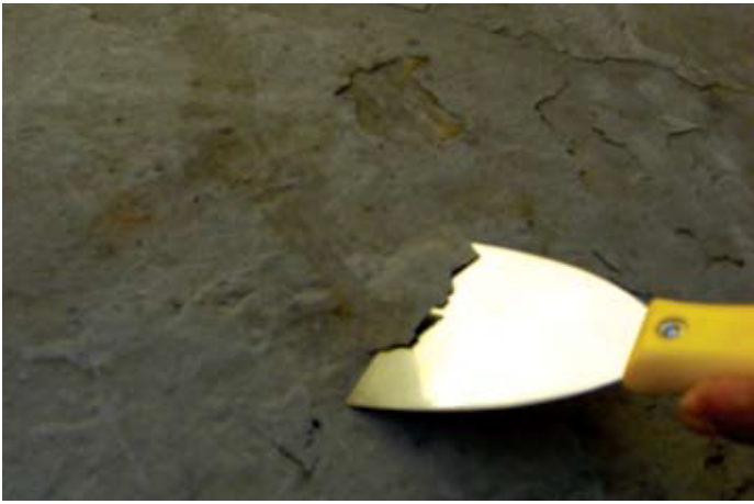
^ Surveyor scraping off loose paint
