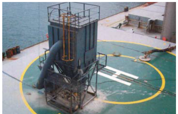
^ Loading cement using a closed loading system
