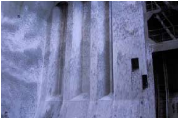
^ Applying the prewash
