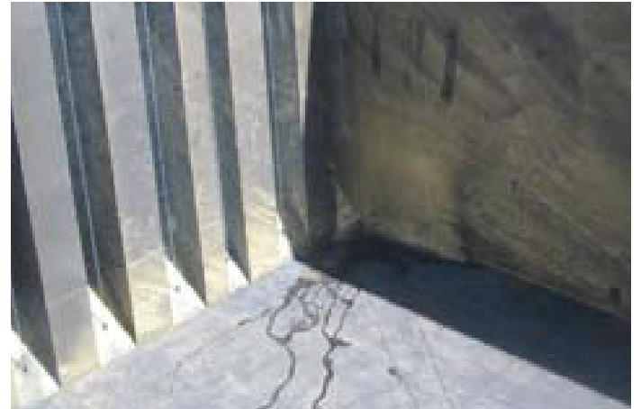
^ Water ingress via a faulty bilge valve will cause cargo damage
