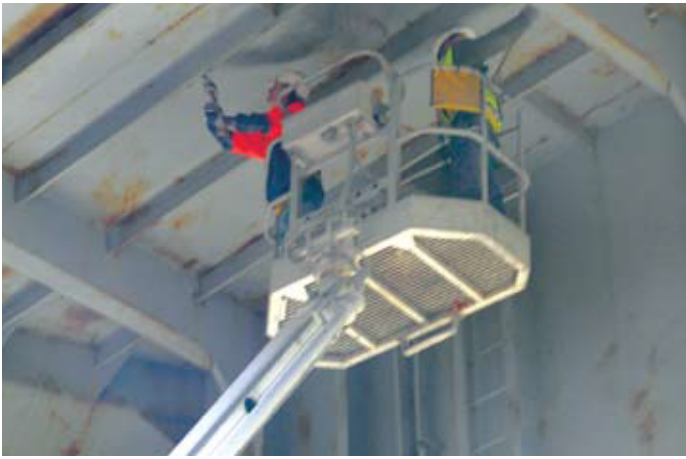
^ Using cherry-pickers to clean the undersides of the holds
