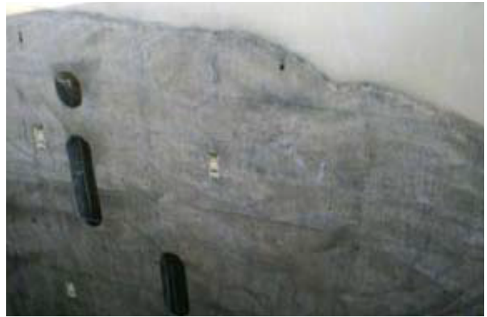
^ Discoloured hold after carriage of petcoke
